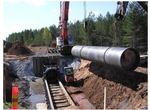
When the drilling is finished, all spirals will be taken out from the sleeve pipe into the starting pit and will be opened one by one. Rest of the equipment will be lifted out from the pit, and inserted pipe will be cleaned again if it is needed. Then the work is finished and it is possible to install desired pipe(s).
